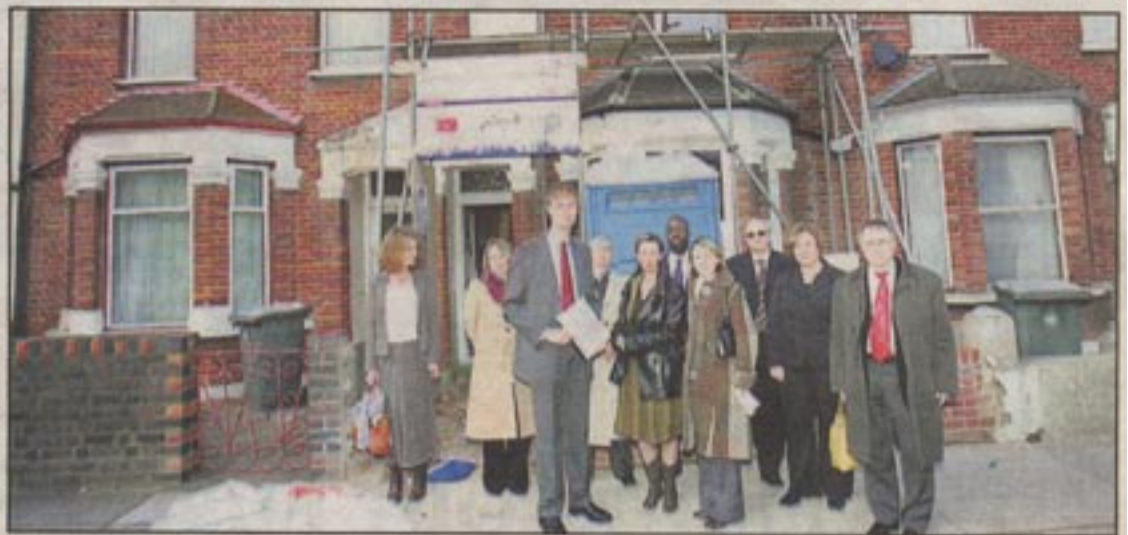
● (Clockwise from above) MP Stephen Timms outside the transformed house with council and housing bosses; the state of the bathroom and kitchen prior to the renovation; Stephen Timms at the launch inside the house
